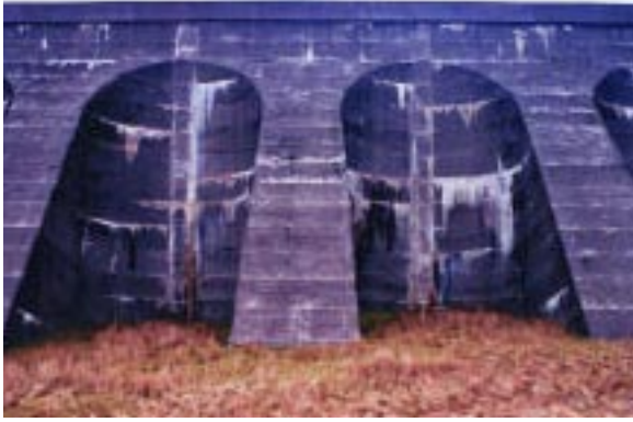
Left: Efflorescence and subsequent spalling on the Stwlan Dam Below: General view of the dam Photos courtesy of the author
