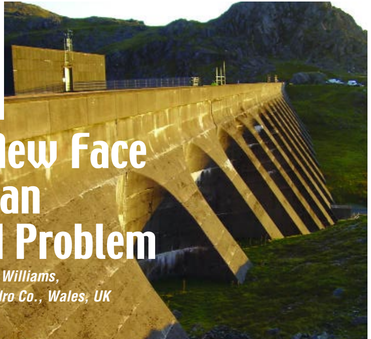
Left: Efflorescence and subsequent spalling on the Stwlan Dam Below: General view of the dam Photos courtesy of the author
